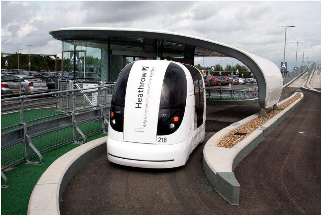
Figure 1. Photograph of PRT vehicle and at-grade station at London Heathrow Airport. PRT vehicles, stations and infrastructure are smaller than typical Automated People Mover and urban rail systems. Vehicle length, width and height are 3.7m, 1.4m and 1.8m, respectively. Photo courtesy of ULTra PRT Ltd.
